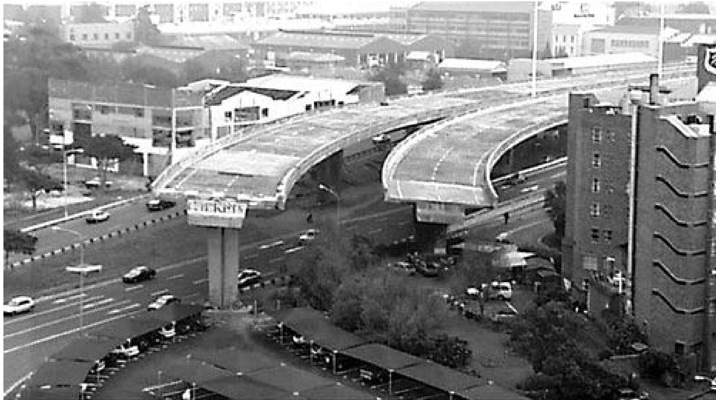
The "Bridges to Nowhere" Cape Town, South Africa
